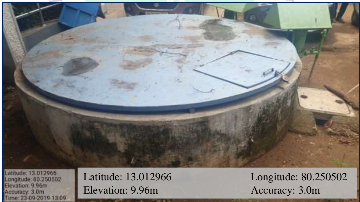
Rain Water Segregation Chamber – D Block
